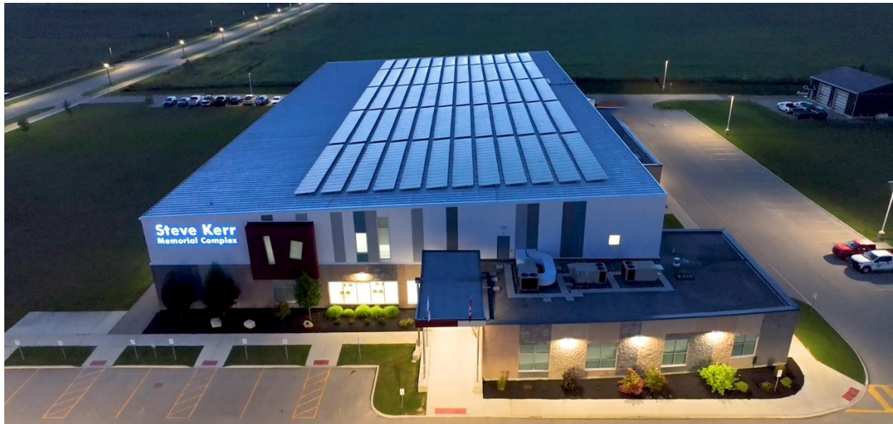
Figure 2 - Solar array at Steve Kerr Memorial Complex
