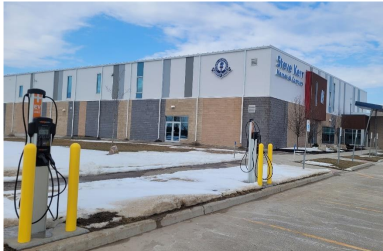
Figure 3 - Level 2 AC Electric Vehicle Chargers at SKMC
