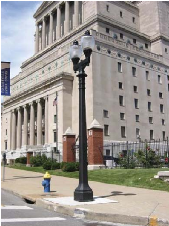
Existing street lighting can be modified to provide more light, for example by using twin headed fixtures.
