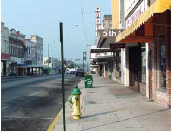
Sidewalk – before pavers added.
