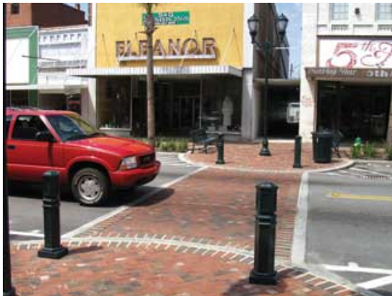
Sidewalk bump-outs and contrasting paving draws drivers' attention to a pedestrian crosswalk. Vertical elements such as bollards can aid visibility in winter.
