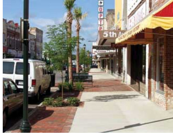
Sidewalk – after pavers added.
