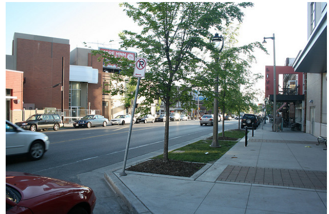
Sidewalk bump-out with trees.
