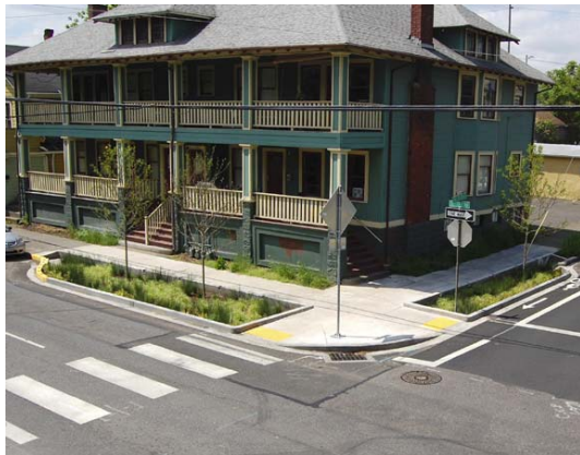
Sidewalk bump-out with trees and low planting.
