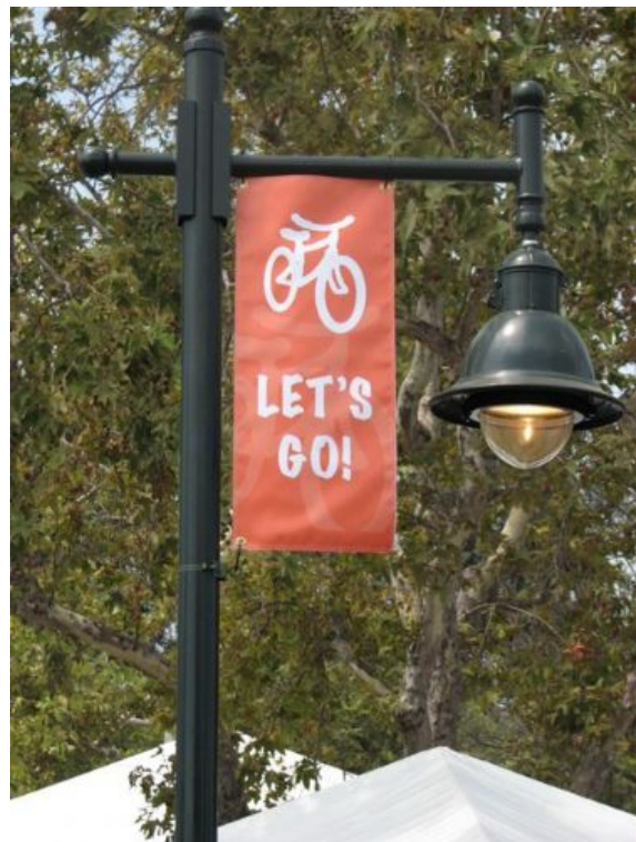
Pendant-style luminaires can be added to increase light in the pedestrian zone. Pendant arms can also accommodate banners or planters.
