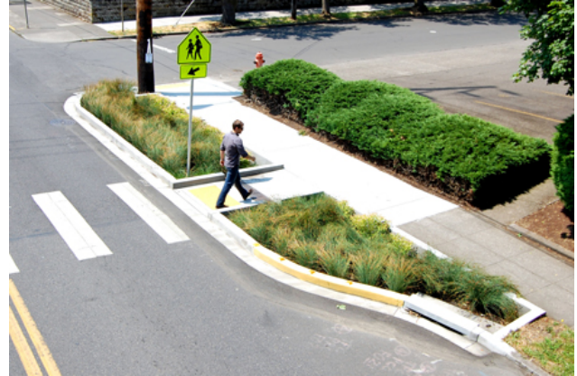
Sidewalk bump-out with plantings and pedestrian crosswalk (Ballard, Washington).
