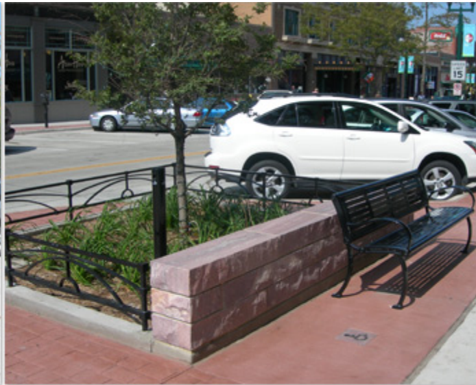
Stone curb and seat wall with decorative fencing.
