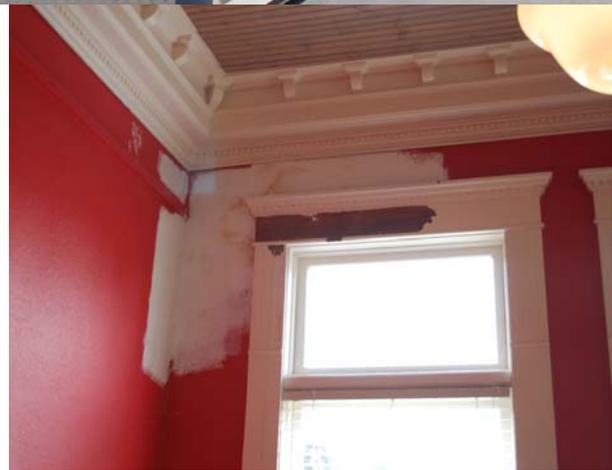
Interior finishes at office, below chimney cricket, have water damaged plaster/gypsum board and staining at wood ceiling.
