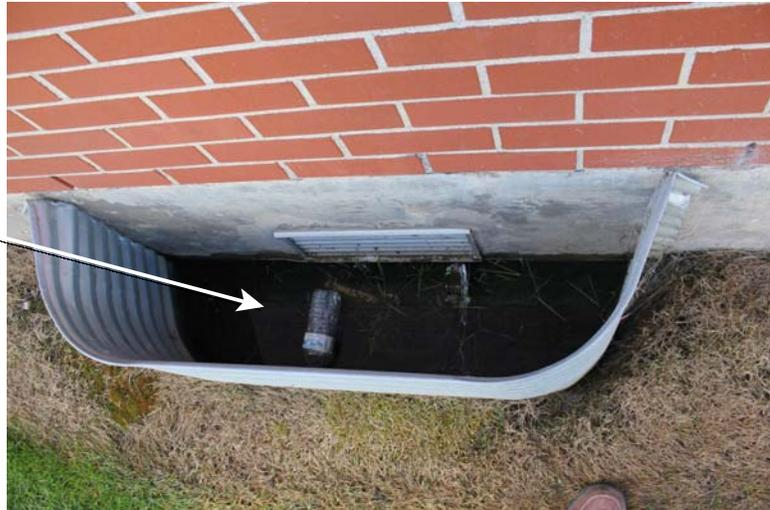
Water staining ran 6" to 12" up the face of the rigid insulation secured to perimeter foundation wall. Water staining is evidence of past flooding of crawlspace.
