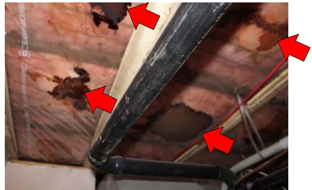
Suspect mould and water staining is visible on top of polyethylene vapour barrier, located above the suspended ceiling system, which is part of the insulated floor assembly between main and second floors. Roof leaks are the likely contributing factor, although, this could not be confirmed because the door to the second floor was secured.
