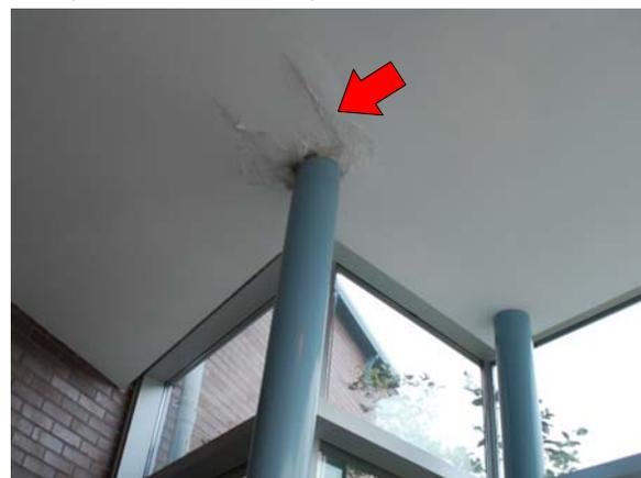
Roof leaks, below scupper (in photograph at upper right), continue to cause damage at interior finishes. Large accumulations of ice are reported to occur during winters, which totally envelopes the exposed, exterior downpipe.
