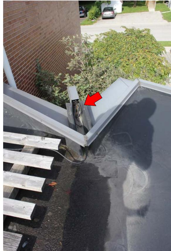
The lobby roof is drained, in part, by a scupper drain in the perimeter curb. Various attempts to prevent water leaks to interior are evident by patches on the EPDM roofing membrane and presence of deicing cable. The wood grating (at left) has been installed to protect the roofing membrane from snow and ice sliding off the metal roofing above.
