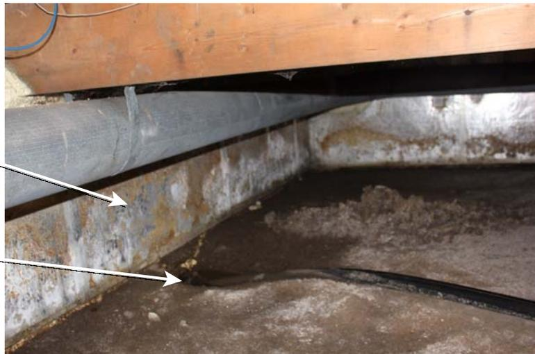
The large rectangular air plenum box in crawlspace is suspended directly below the main floor furnace. Staining and rusting at bottom 4" of plenum box records elevation of previous water accumulation in the crawlspace. Furnace air, flowing over uncontrolled water source, is a health concern.
