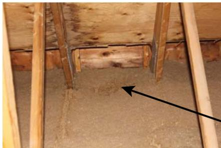
Leaks from uppermost roof have caused damage to walls and ceilings below.
