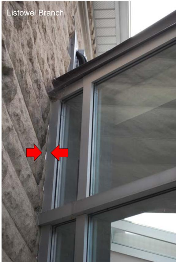
The aluminum/glass wall at courtyard intersects the south masonry wall of the original Carnegie Library building at an angle. This interface appears to rely heavily on caulk sealant and it has been a persistent source of water leakage since construction.
